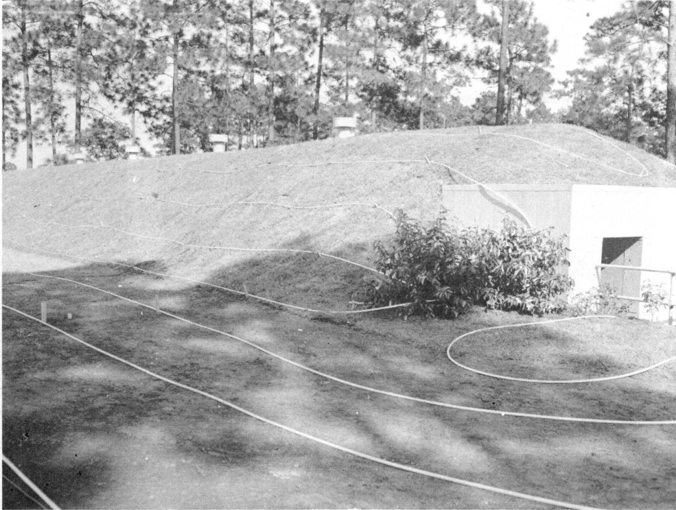
Fig. 2.13—Tubing layout at shelter.
